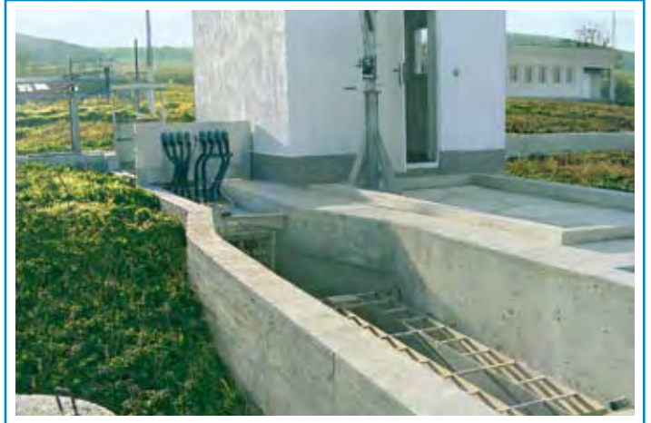
WWTP, Beloslav, Bulgaria, 20 400 m 3 /day
