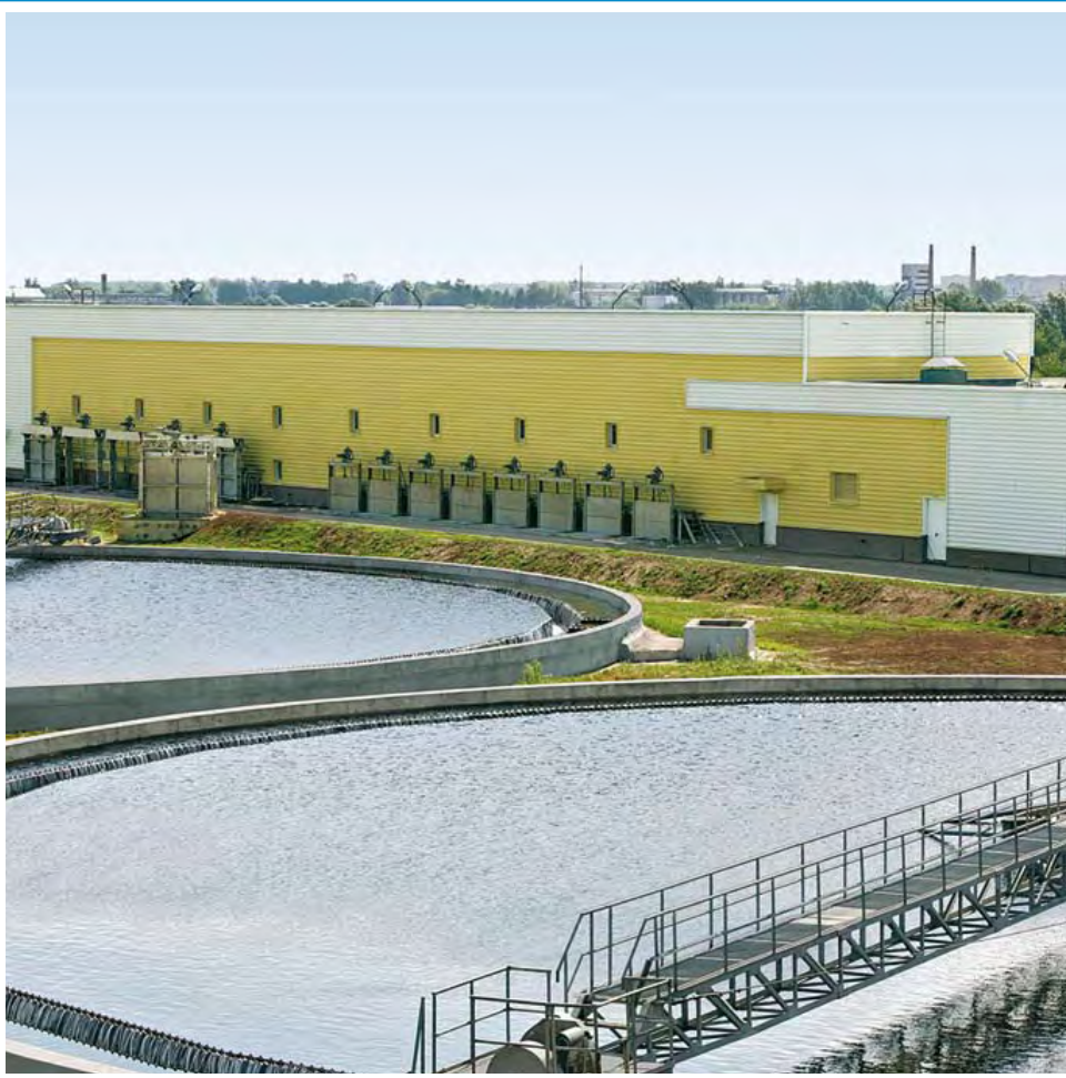
Luberetskiye WWTP, Moscow, Russia, 1 350 000m 3 /day
