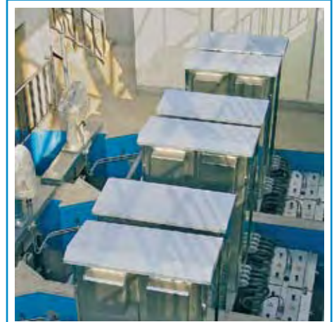
WWTP, Gumi, South Korea, 330 000 m 3 /day
