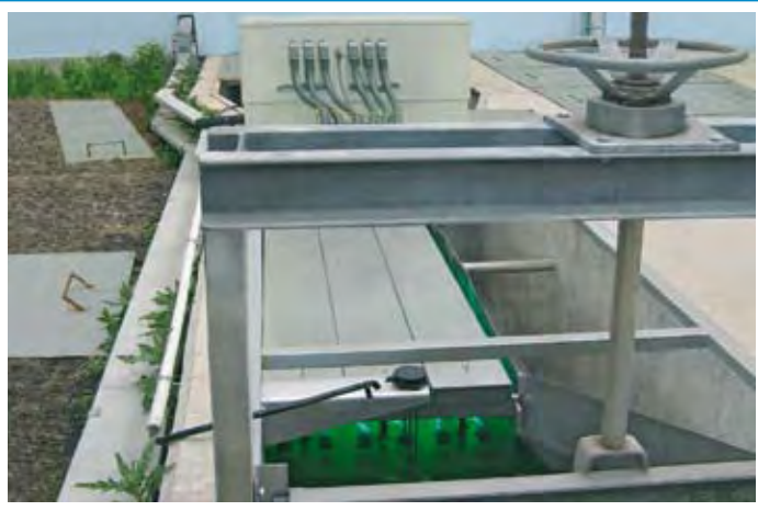
WWTP, Usak, Turkey, 20 400 m 3 /day
